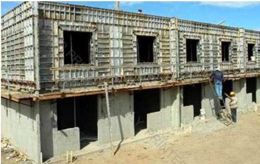
Formwork before concrete pouring
