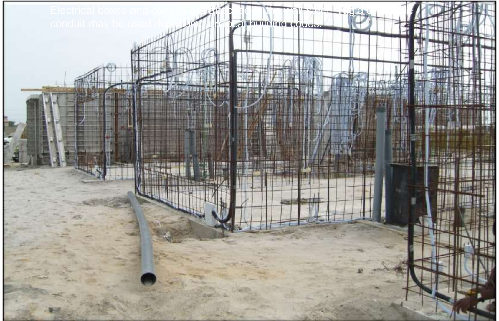
The passage of electrical ducts and plumbing before formwork
