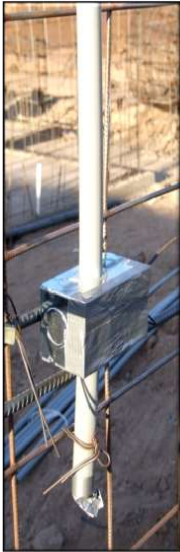
The passage of electrical ducts and plumbing before formwork
