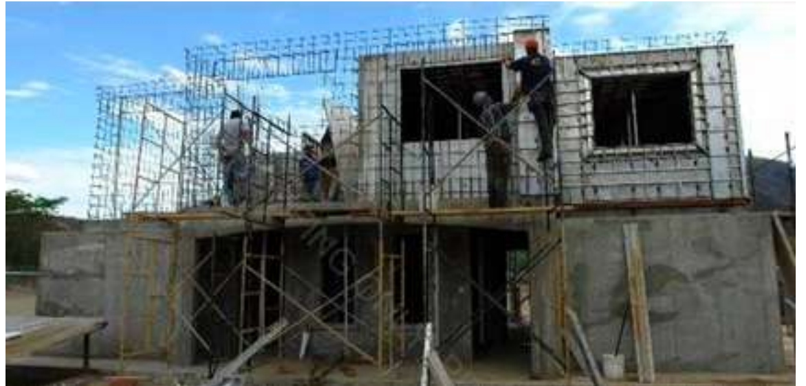
Formwork before concrete pouring
